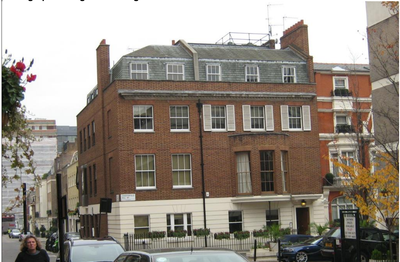
Photograph 1: Original building before demolition
